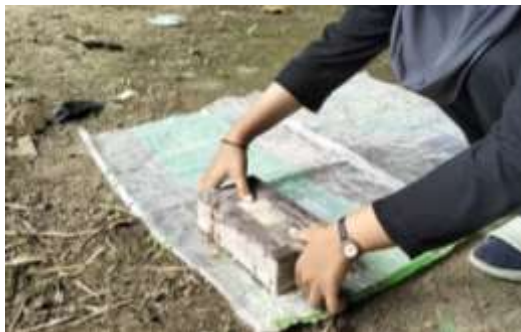
Proses Pencetakan Paving Block
