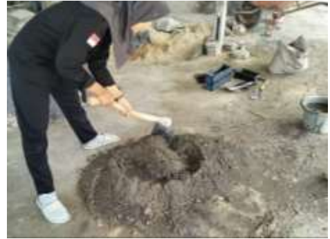
Proses Pengadukan Bahan Paving Block
