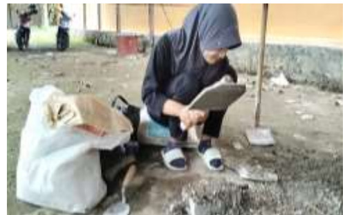
Proses Pemadatan Paving Block
