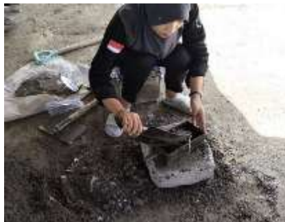
Proses Pencetakan Paving Block
