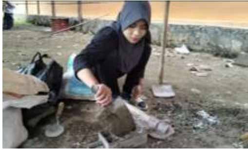
Proses Pemadatan Paving Block
